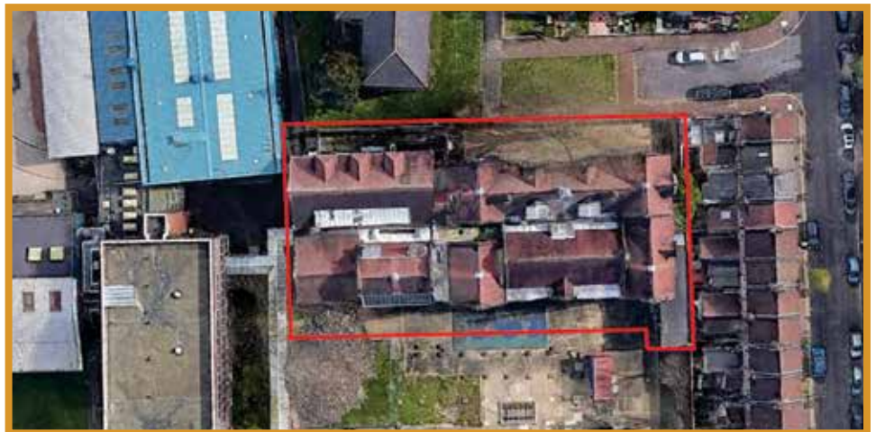
Aerial View, with red lines indicating the approximate boundary
